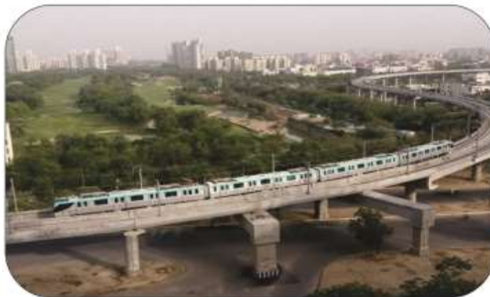
Project of Metro connection between Noida and Greater Noida (29.707 km) [Estimated Cost – Rs. 5503 Cr; Loan Sanctioned – Rs. 1587 Cr.]
